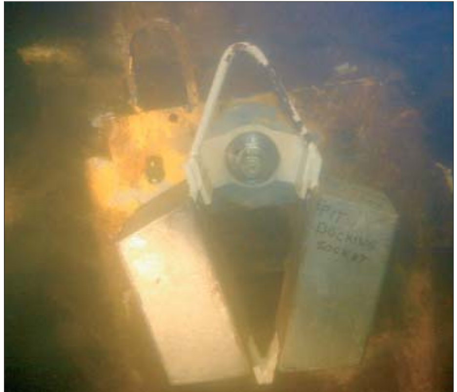
Anode mounted on PIT clamp 15 on Troll B.
