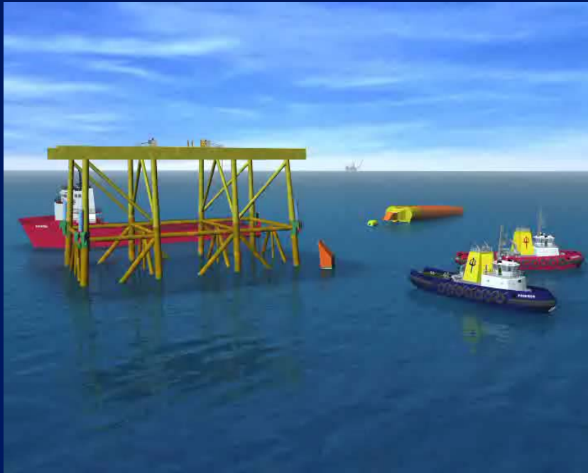
One tank moored while the first one is installed.
