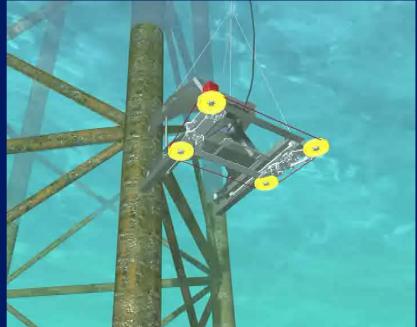
Diamond wire cutting (in figure above represented by Tecnospace DWC)
